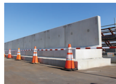
既設防潮堤(2.4~4.2m)
