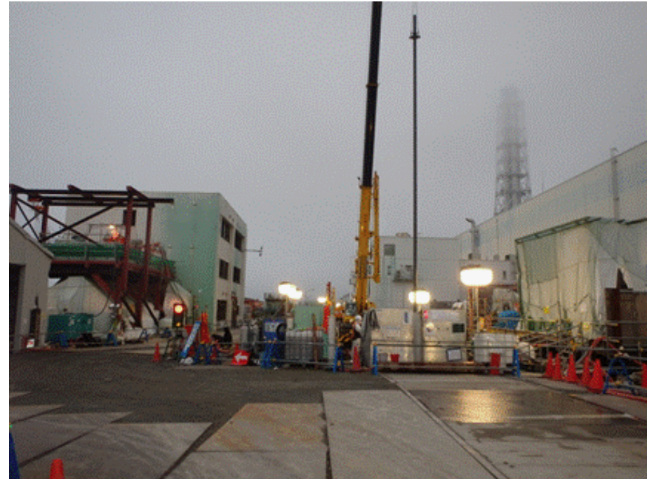
写真⑪-2 11BLK凍結管建込
