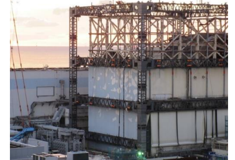
(Dismantling of Unit 1 building cover wall panels)
