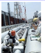
(Opening/closure of frozen pipes)
