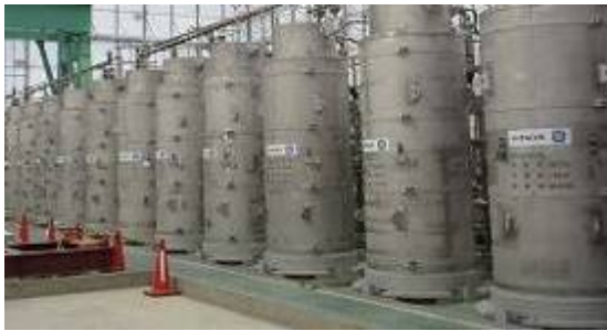
Figure 3: High-performance multi-nuclide removal equipment (ALPS)
