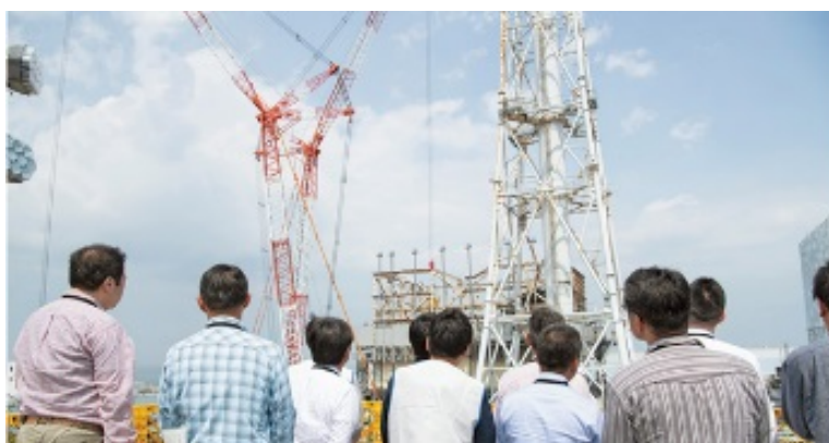
Figure.9 Site visit without wearing protective clothing
