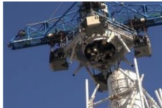
Figure 5: Dismantling of exhaust stack of Unit 1/2 (Started in August 2019)
