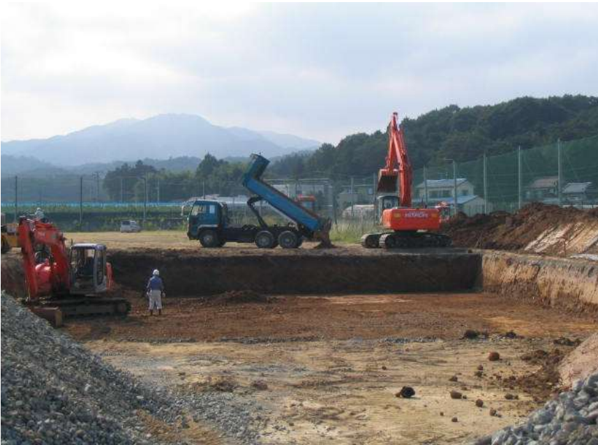
Replacement of soils
