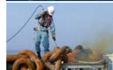
Mooring of the floating structure of the wind turbine: the work was implemented both on and under the sea while adjusting the angles carefully. The mooring chains weigh as much as 330 tons per chain.
