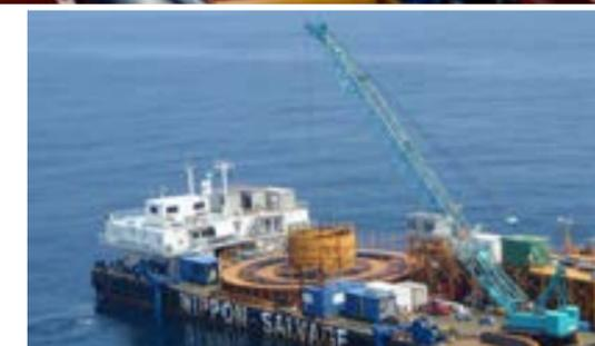
A cable to connect floating structures that move one another, which was developed by Furukawa Electric Co., Ltd. and VISCAS Corporation, was laid through the joint venture. New achievements were made one after another, such as succeeding in the difficult work of drawing in the cable to the bottom of the floating structure.
