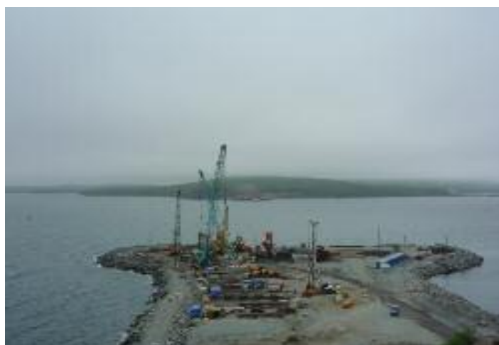
Construction site of a bridge to Russky Island
