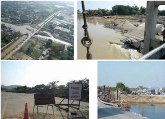
Figure 2-3-1-8 Burst of floodgates by last year’s flood in Thailand (above) and highways with breached levees (below)
