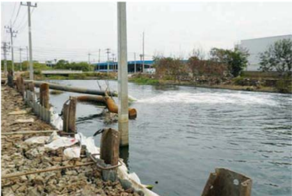
(Right) discharge of floodwater from the broken embankment at the Rojana Industrial Estate (continued after the completion of the discharge of the industrial estate).
