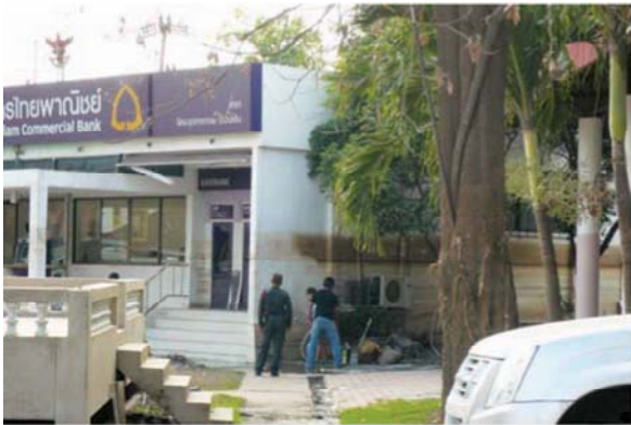
Source: (Left) near the front gate of the Bang Pa-In Industrial Estate (workers cleaning up the aftermath of flooding). Pictures taken by METI (December 15 (left) and 16 (right), 2011).
