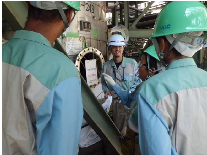
OBSERVED OPEN MAINTENANCE
