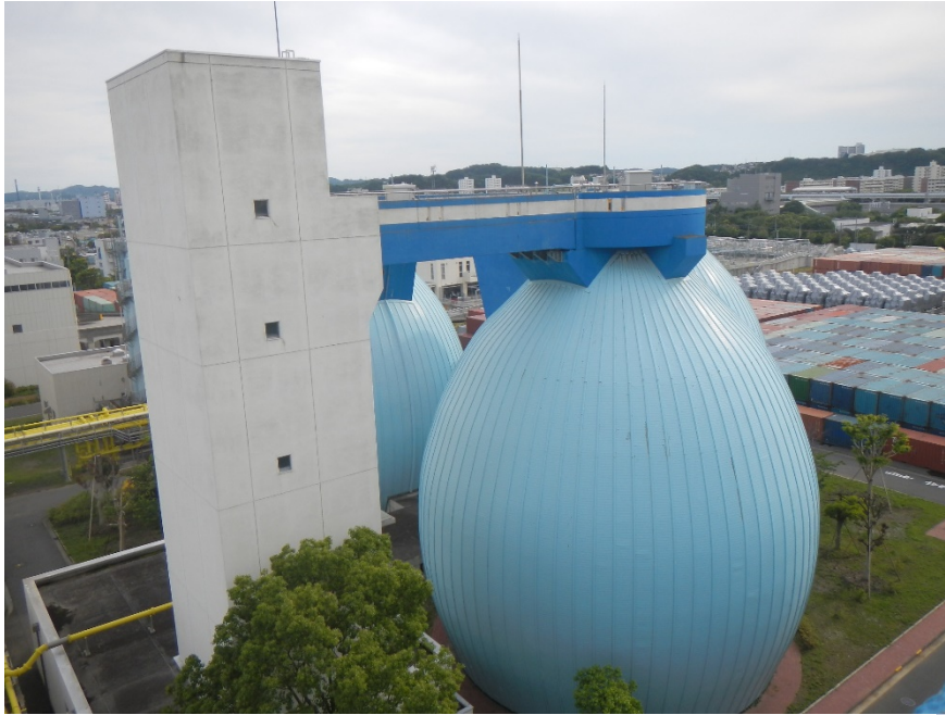
Egg-Shape Sludge Digester
