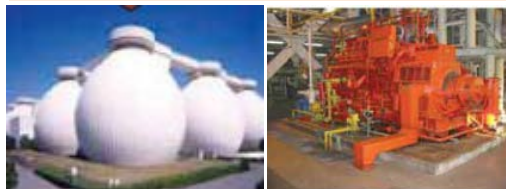
Sludge treatment and energy recovery
