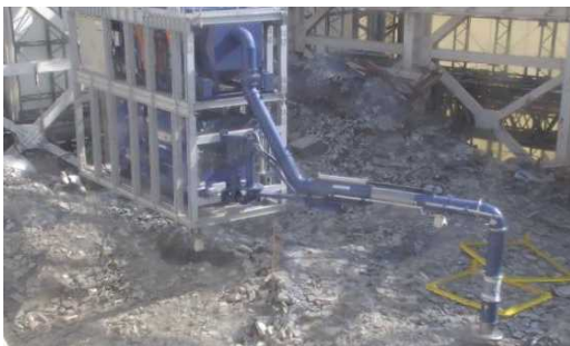
©Tokyo Electric Power Comp. 小ガレキ吸引装置 rved.
