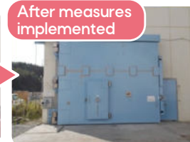
Installation of watertight Doors
