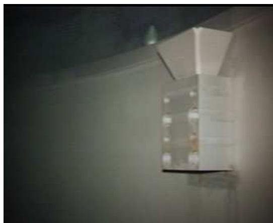
Core shroud stand (bottom of RPV) after decon at Unit 2
