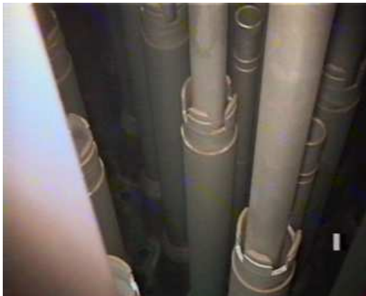
CRD Housings (bottom of RPV) after decon at Unit 2
