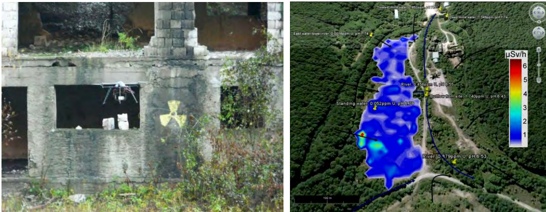
Images of (left) the ARM system in flight at an abandoned radiologically contaminated building in Romania and (right) site radiation dosimetry survey data.
