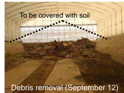
7. Debris storage in the temporary waste storage facility (Soil covering type)
