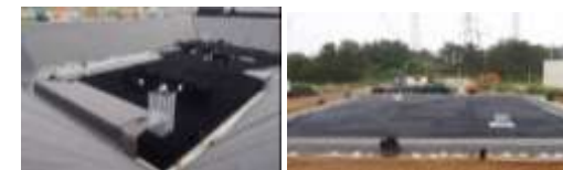
Underground water storage tank installation
