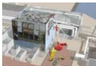
Debris removal from the upper part of the Reactor Building
