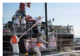
Unused fuel being taken out at Unit 4 spent fuel pool (July 18-19)
