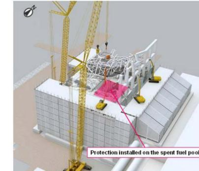
4. Simulated image of Unit 3 debris removal
