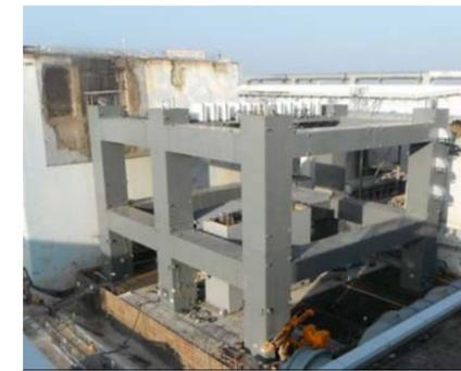
3. The second layer of the steel frame completed (Photo taken on February 28)
