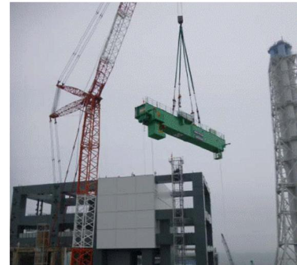
Figure 5: Lifting of overhead crane for Unit 4
