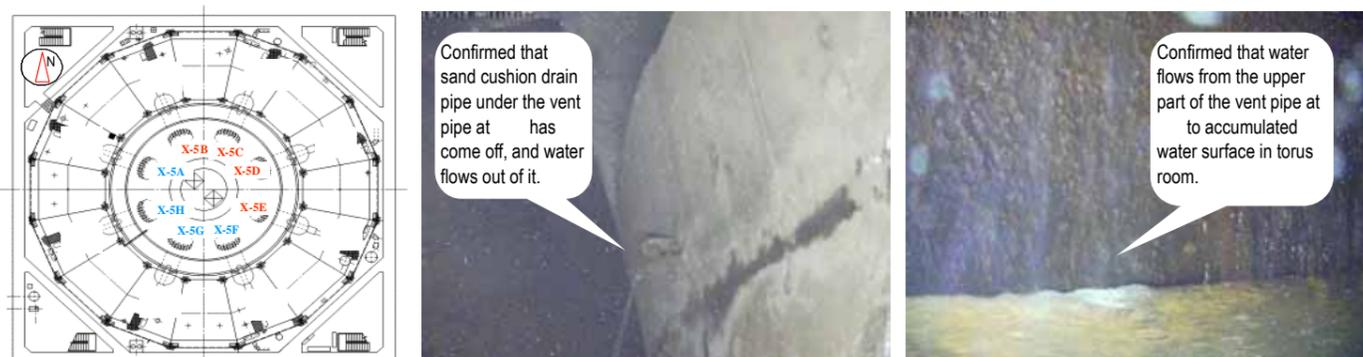
Figure 8: Water leakage from sand cushion drain pipe and upper part of vent pipe at Unit 1
