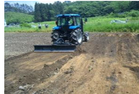
Removal of topsoil
