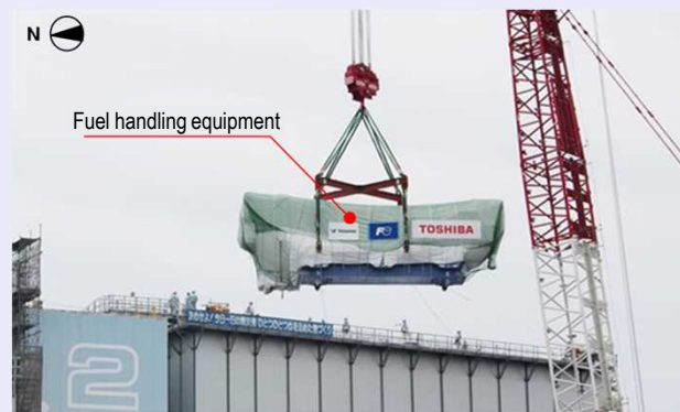
Fuel handling equipment being hoisted (outside) on May 30, 2025
