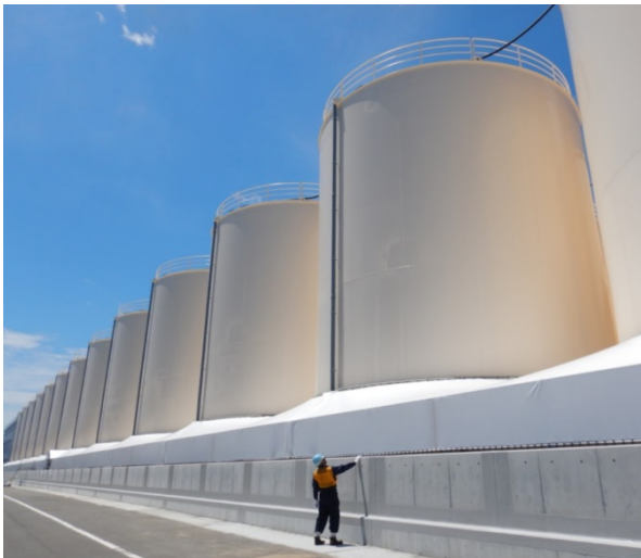
Tank groups storing treated water
