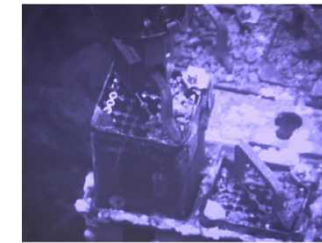
Removed fuel (assemblies)
