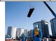
Construction of welded-joint tanks
