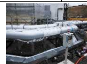
Land-side impermeable wall brine (refrigerant) circulation pipe
