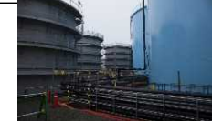
Flanged and welded-joint tanks
