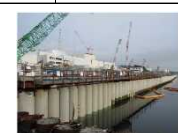
Placement of seaside impermeable walls complete
