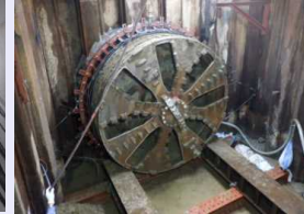
<(2) Upstream side propulsion pipe reached>
