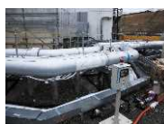
Land-side impermeable wall brine (refrigerant) circulation pipe
