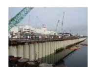
Placement of seaside impermeable walls complete
