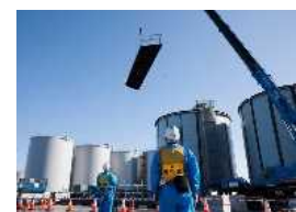
Land-side impermeable wall brine (refrigerant) circulation pipe
