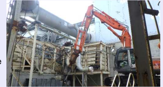
<Rubble removal work>
