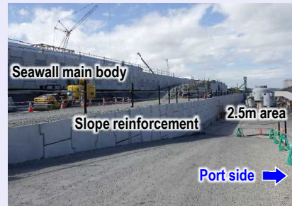
<Construction of the seawall main body>
