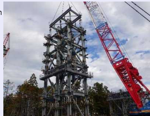
<Steel frame unit connection verification (November 5, 2022)>
