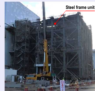
< Work on the south side of Unit 2 Reactor Building > (August 10, 2023)
