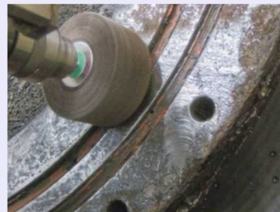
< Cleaning of X-6 penetration flange surface >
