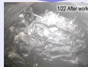
< Deposit removal by low-pressure water >
