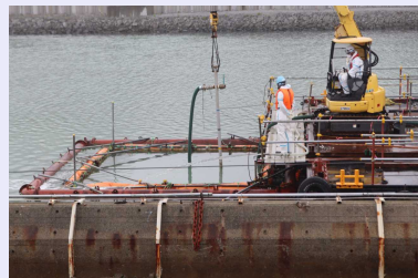
< Seafloor re-covering construction (layer of cover) >
