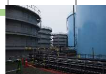
Flanged and welded-joint tanks
