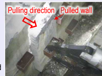
<Work to pull down the wall>
