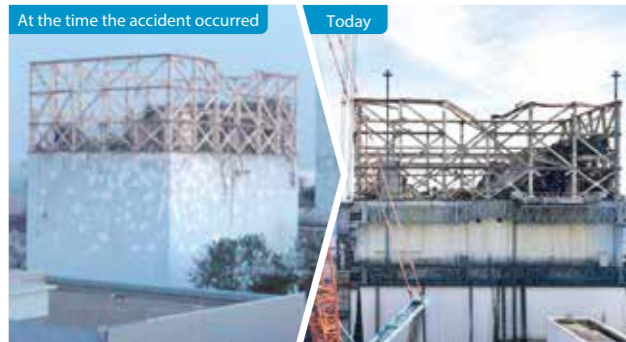
A cover that is large enough to spread over the entire building will be installed to prevent dust scattering during planned fuel removal.
