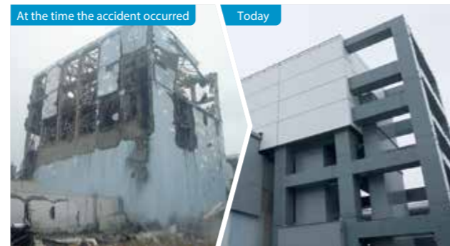
All fuel assemblies have been removed and transferred to the common pool or other places, and they are stored and managed safely.
