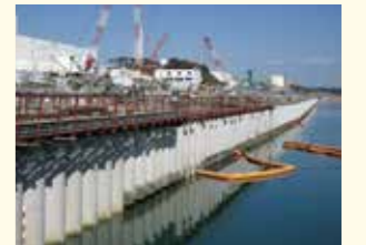
Sea-side impermeable wall
