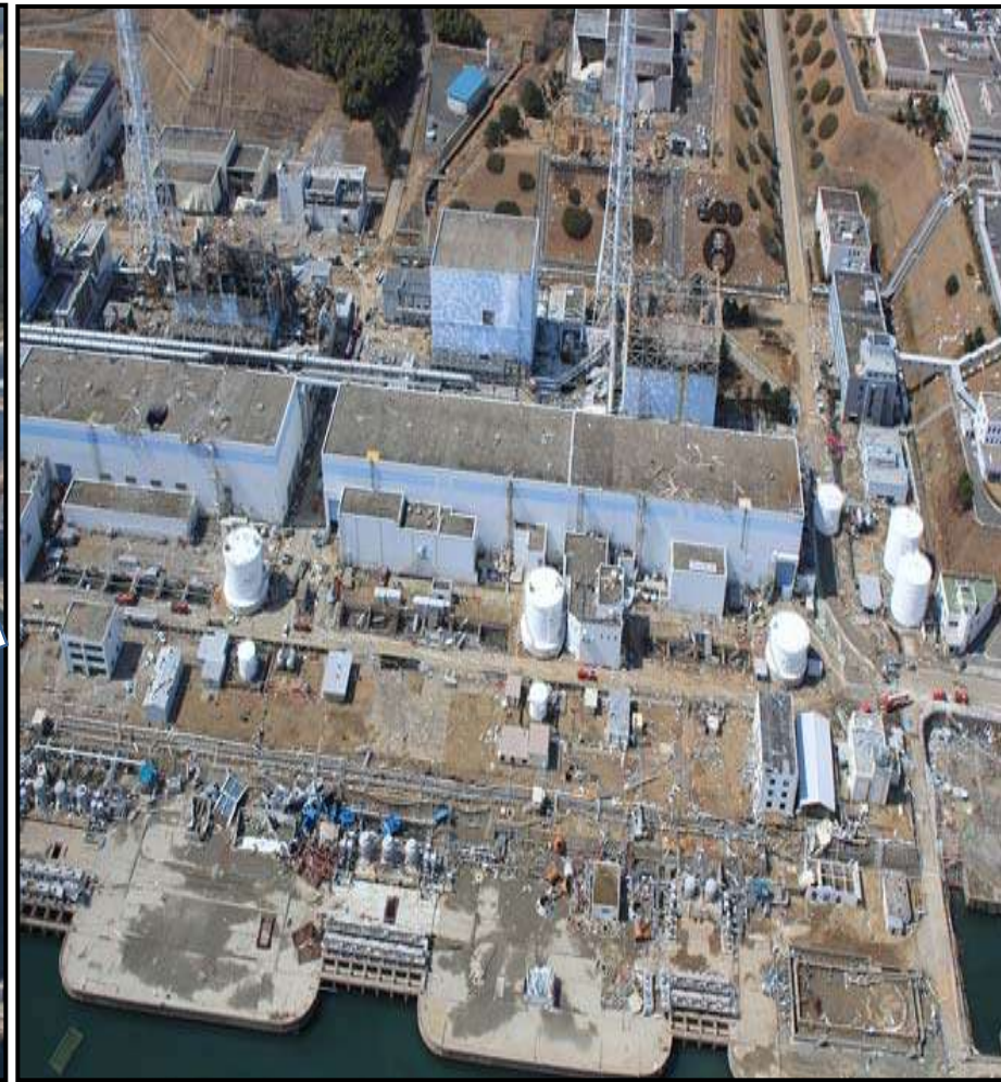
After the Earthquake and Tsunamis
