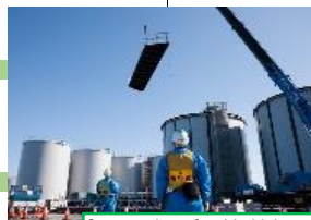
Construction of welded-joint tanks
