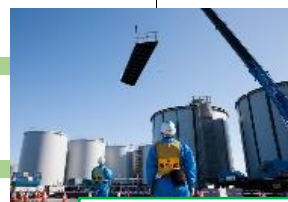
Construction of welded-joint tanks
