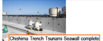
Chishima Trench Tsunami Seawall complete
