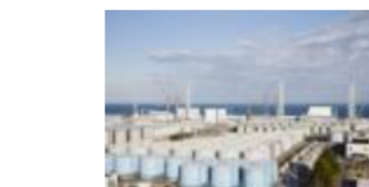
Tank area viewed from the Large Rest House (2015.10.29)
