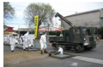
Removal of sludge in the ditch at Namie Town office
