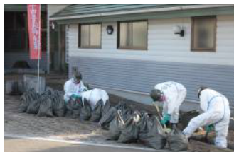
Removal of sludge in the ditch at Iitate Village office
