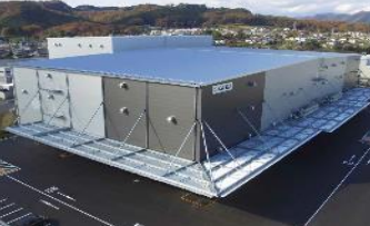
Mitsui Foods Distribution Center
