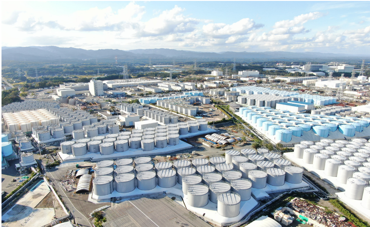
Figure 1.2. Storage tanks for contaminated water at FDNPS
