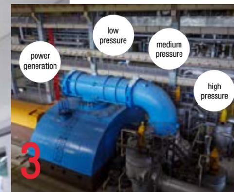
3 The jet and expansion forces of the steam transmitted to the turbine turn the blades at high speed. As the generator rotor turns, electricity is generated.
