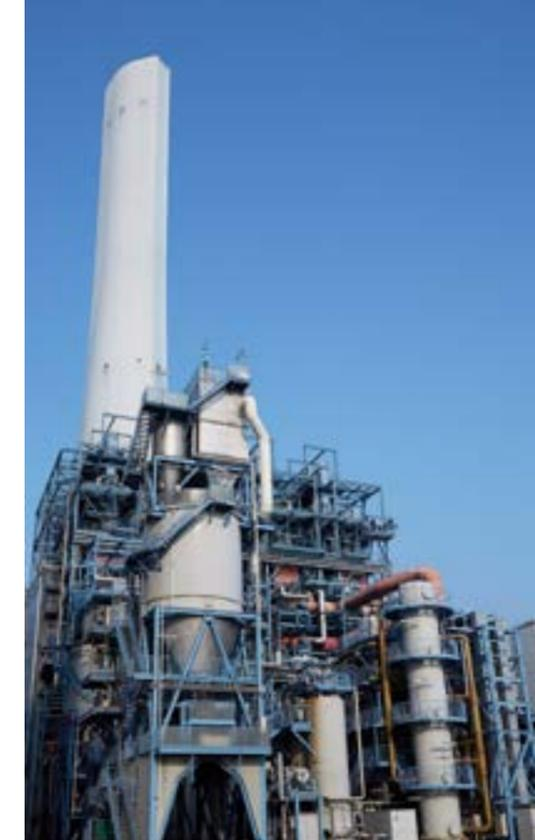
Dry-type desulfurization equipment uses activated coke created from coal to absorb SOx contained in exhaust gas. The activated coke is recycled.
