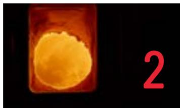
2 Isogo Thermal Power Plant is the first power plant in Japan to use a tower-type boiler. Inside the boiler, the temperature reaches 1,300 degrees Celsius. Water flowing through thousands of narrow pipes is heated to generate high-temperature, high-pressure steam.
