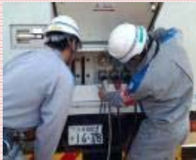
(Recovery of power using power source cars and resumption of power supply)
