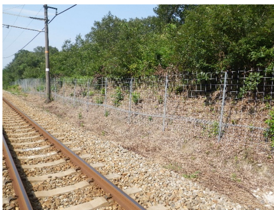
Figure 4-20 Mesh Fence
