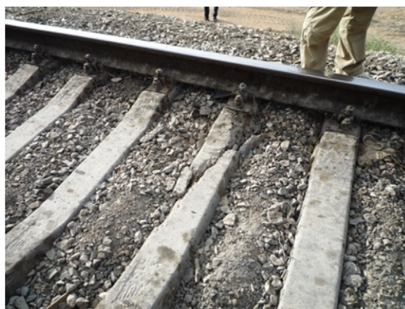
Figure 3-13 Damaged Sleeper
