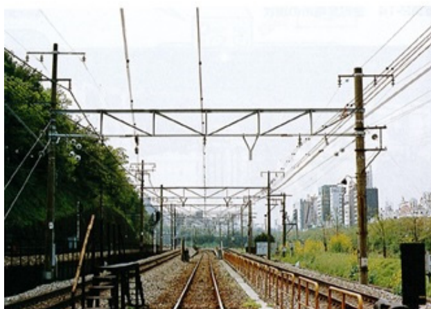
Figure 4-31 Overhead Catenary Line
