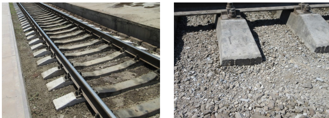
Figure 3-11 Lack of Ballast
