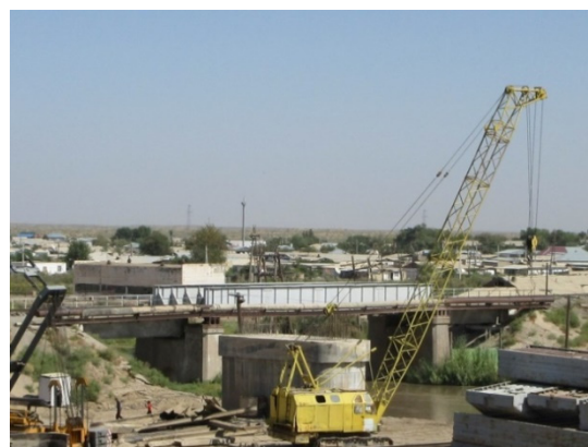
Steel Through Plate Girder
