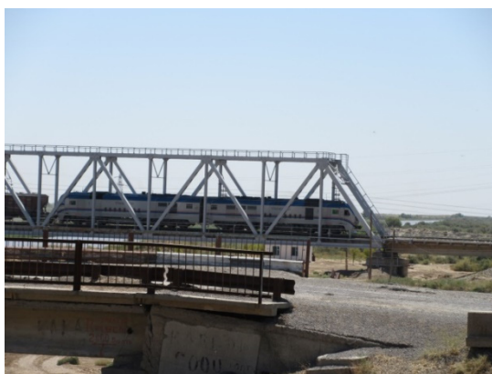
Steel Through Truss Girder
