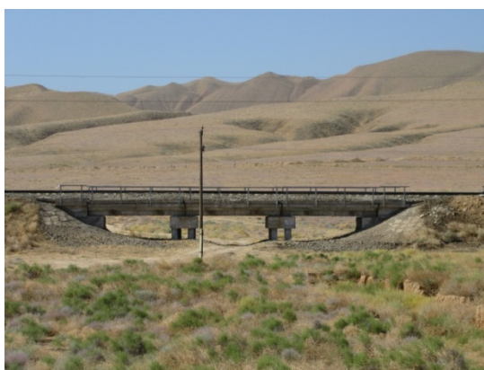
Reinforced Concrete Girder
