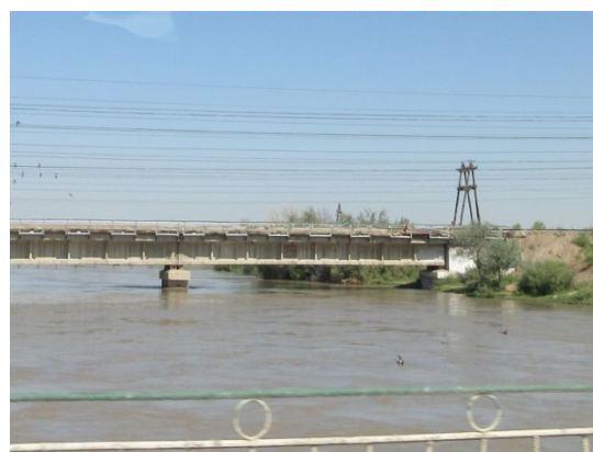
Pre-stressed Concrete Girder
