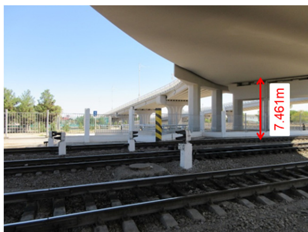
Figure 3-20 Clearance under the Overpass near Ashgabat Station
