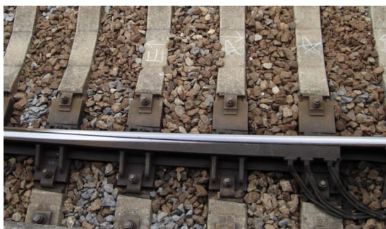
Figure 4-27 Joint Structure for Continuous Welded Rail in Japan
