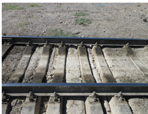
Figure 3-10 Roadbed Mud-pumping
