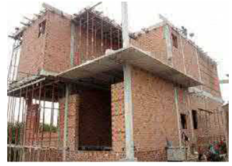
House under construction. Walls are brick.
