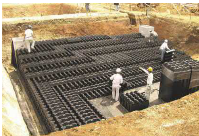
▲ Installation of CROSS-WAVE
