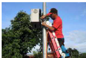
▲Installation of Alarm Unit (City of Iloilo)
