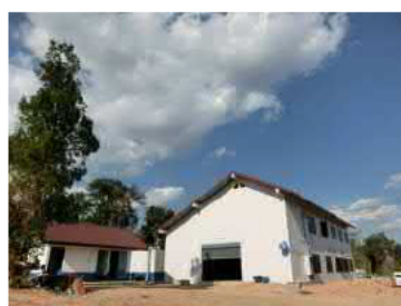
▲Paksan district water purification system building
