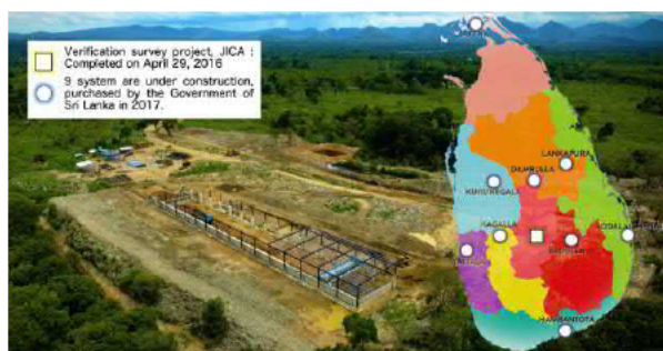
▲ 9 system are under construction
