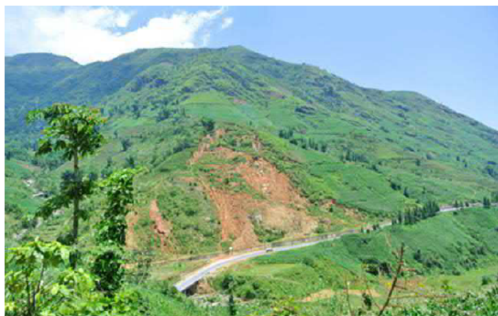
▲Local situation where measures for landslide prevention is required
