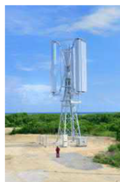
◀ Magnus x Vertical Axis Wind Turbine 10kW Prototype (Ishigaki City, Okinawa)
