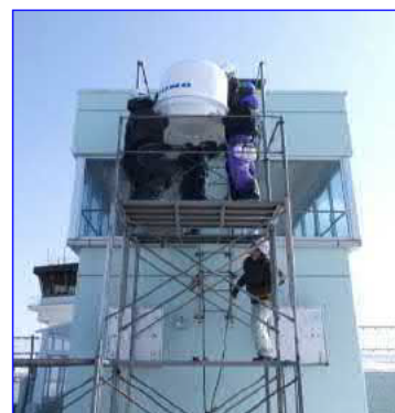
Compact size enable to install on top of existing building and to save costs and period for installation
