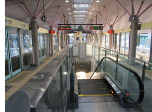
Example of platform (Yurikamome : Shiodome Sta.)
